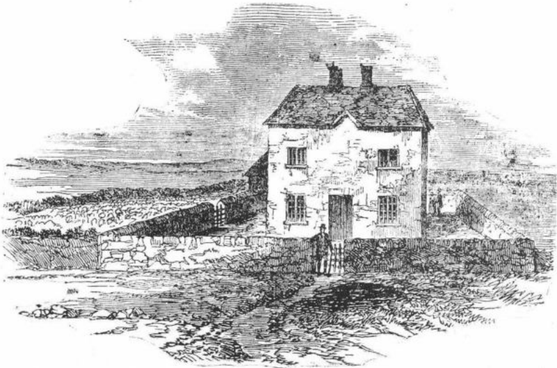
The War House near Ballingarry, County Tipperary
