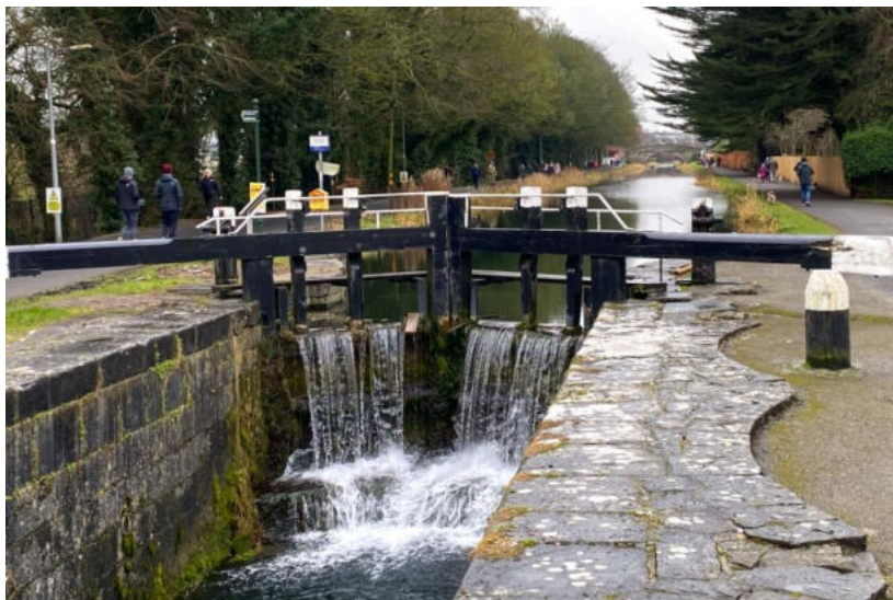
The 5 th Lock, Abbey Bridge with walkers on the canal bank. The solid stone base is visible below lock gates
