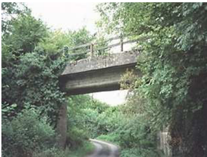
A bridge which carried the railway over a road near Kilfeacle
