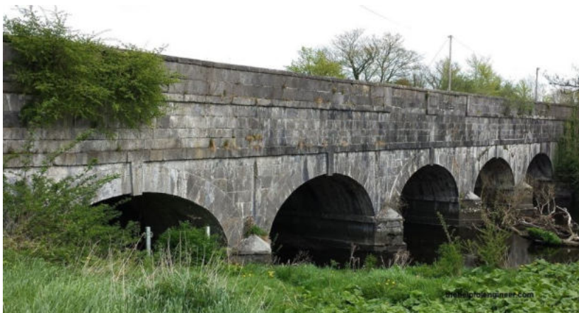
The Leinster Aqueduct
