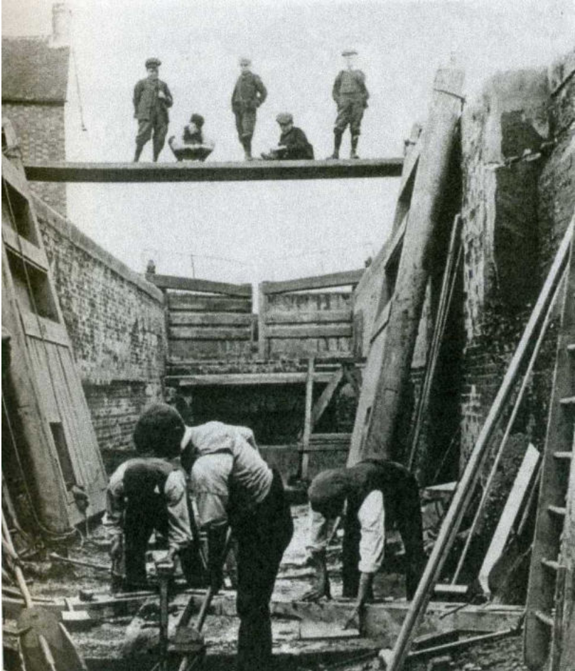
Repairing a lock
