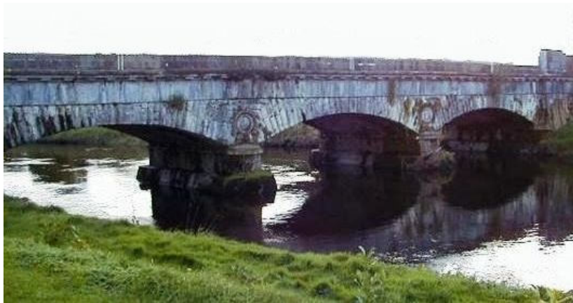
The Barrow Aqueduct Monasterevin built 1826
