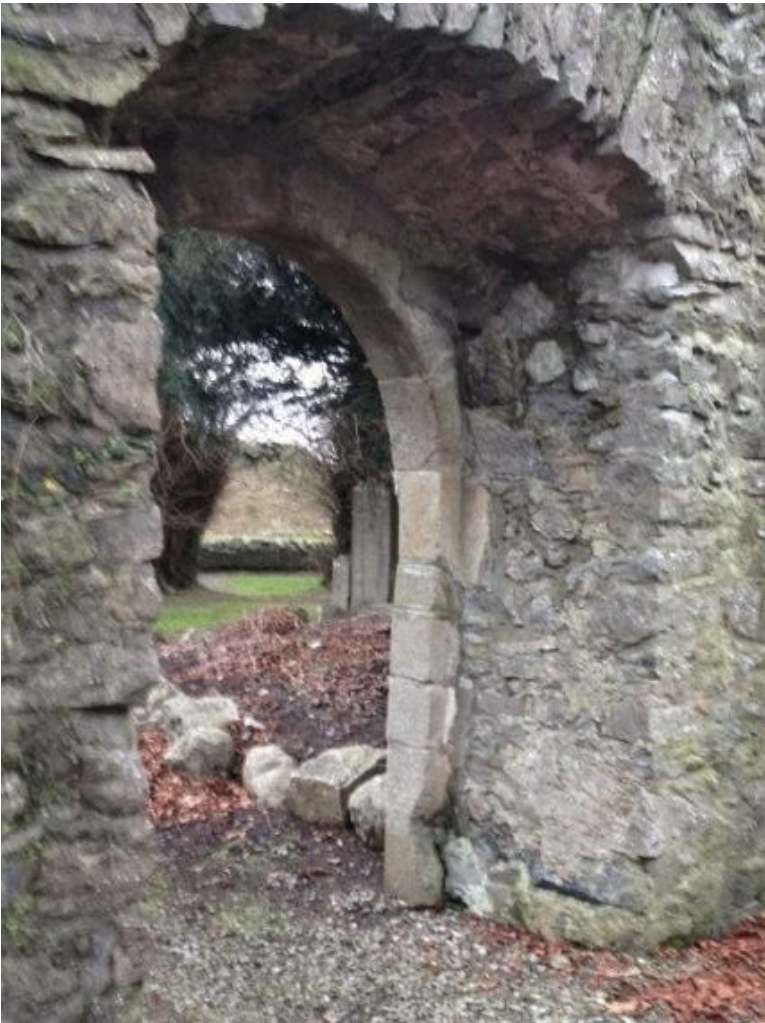
A view through the doorway of Mainham church ruins showing the Motte in the background – notice also the very substantial wall thickness.
