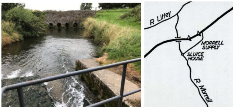
The aqueduct carrying the canal over the Morrell river. The photograph was taken at the spot where water is diverted to the Morrell supply which enters the canal after it descends through the 14th and 15th locks
