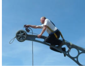
Priming/painting the crane
