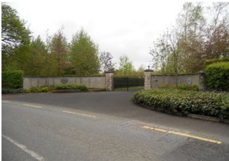
Blundell House entrance, Millicent, Clane
