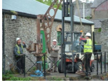
Waterways team assemble crane
