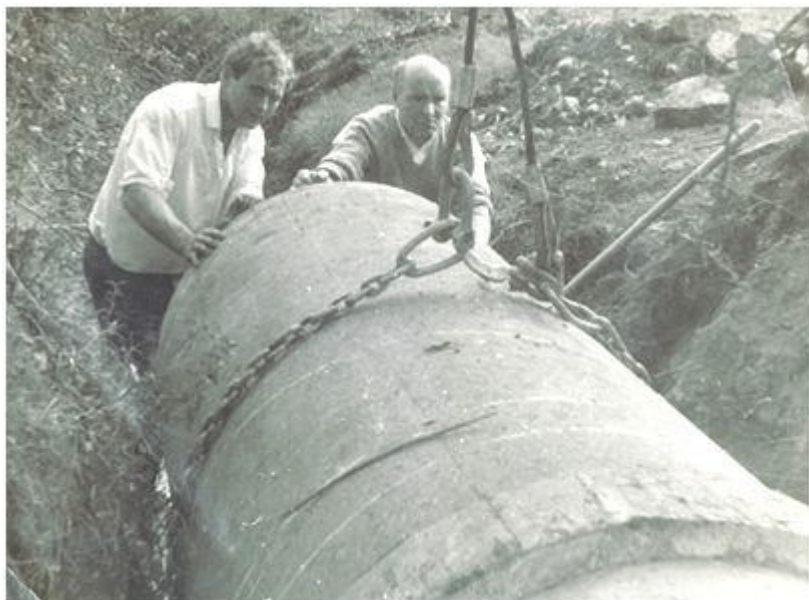
The late Sean Cribben and J. J. Langan position one of the drainage pipes.: courtesy of the Cribben family.
