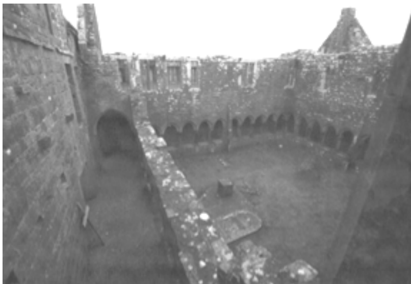
Example of Cloister abutting wall of friary as is suggested for Clane
