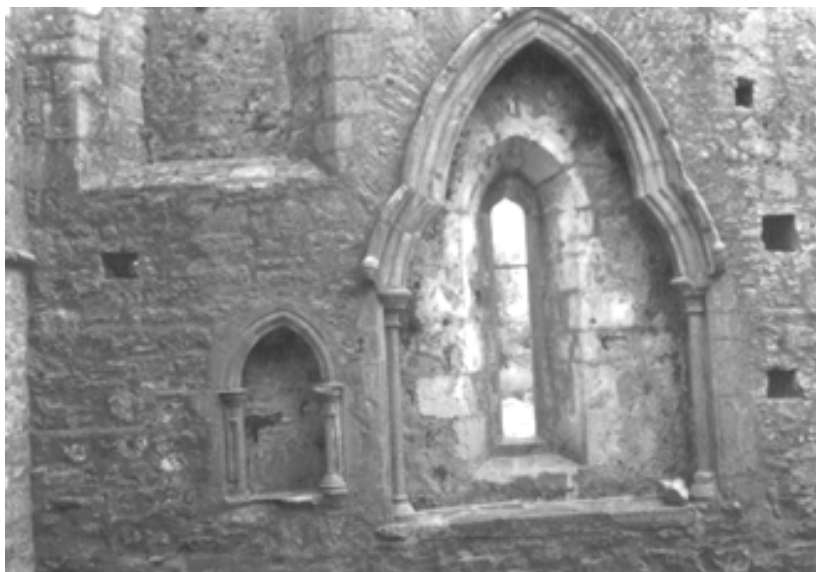
Example of sedilia and piscina in the interior of a Franciscan church
