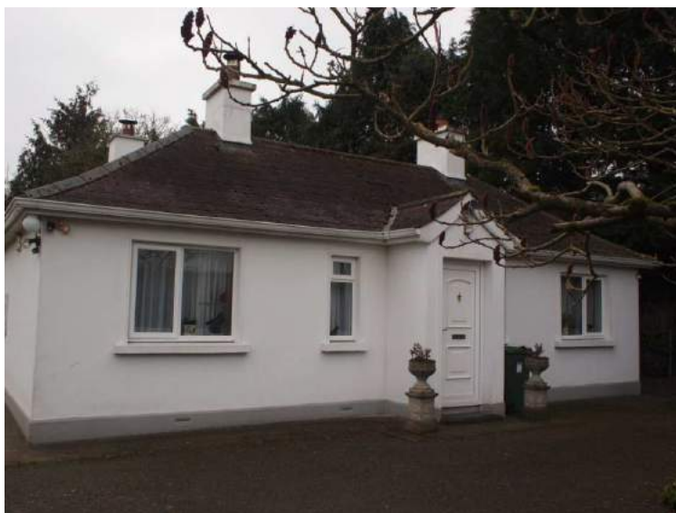
The former Jubilee Nurse's Cottage at Firmount
