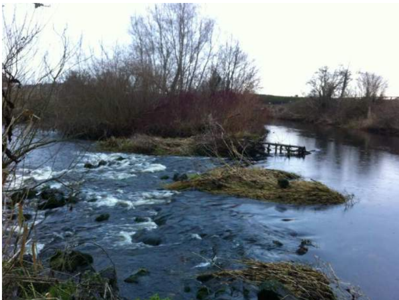
The weir from the left bank. The middle is covered with vegetation
