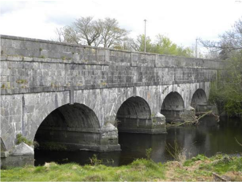
The River Liffey flowing beneath the Leinster Aqueduct
