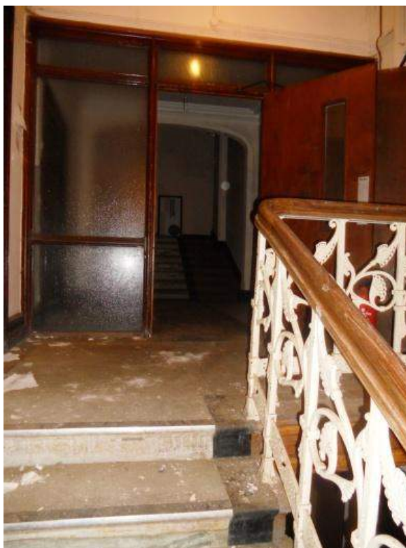
A view of some internal modifications to convert Firmount House into a sanatorium
