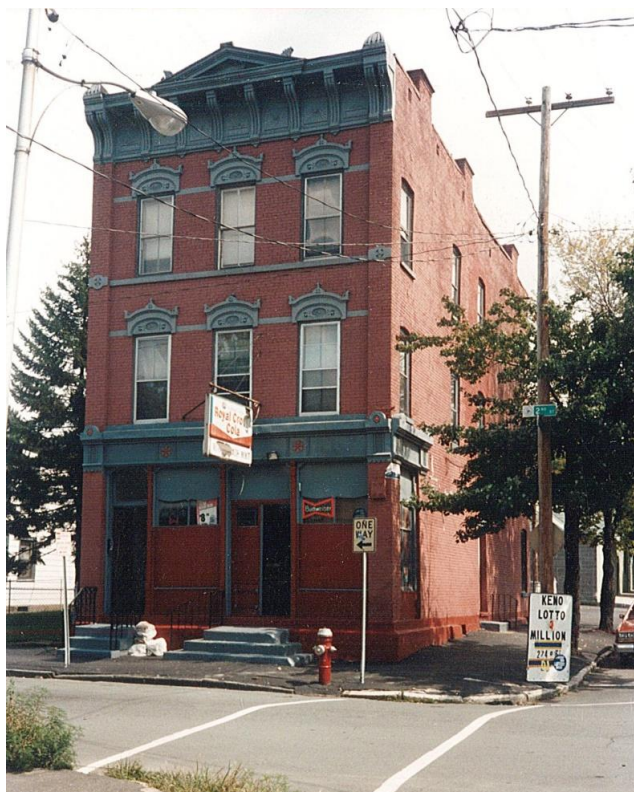
The building in Troy where the Dunn family lived and operated a grocery store for many years
